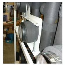
• With gasket in place on each header of the positioned unit (see Figures 9 and 10), move the second module into position and line up the piping. Ensure alignment is maintained for any additional modules to be added.
