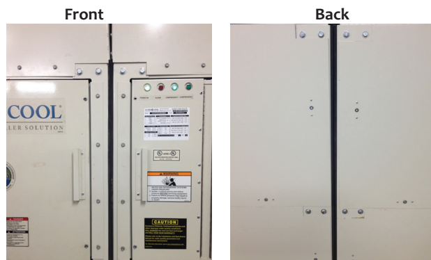
Figure 8: Gasket Installation Between Modules
