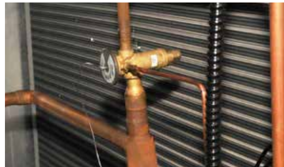
Figure 40 - Expansion Valve
