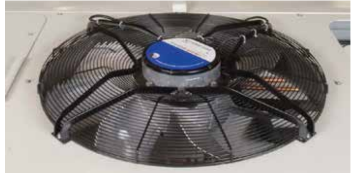
Figure 31 - Variable Speed EC Condenser Fan
