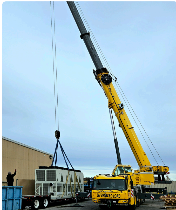
Pre-piped skid being installed
