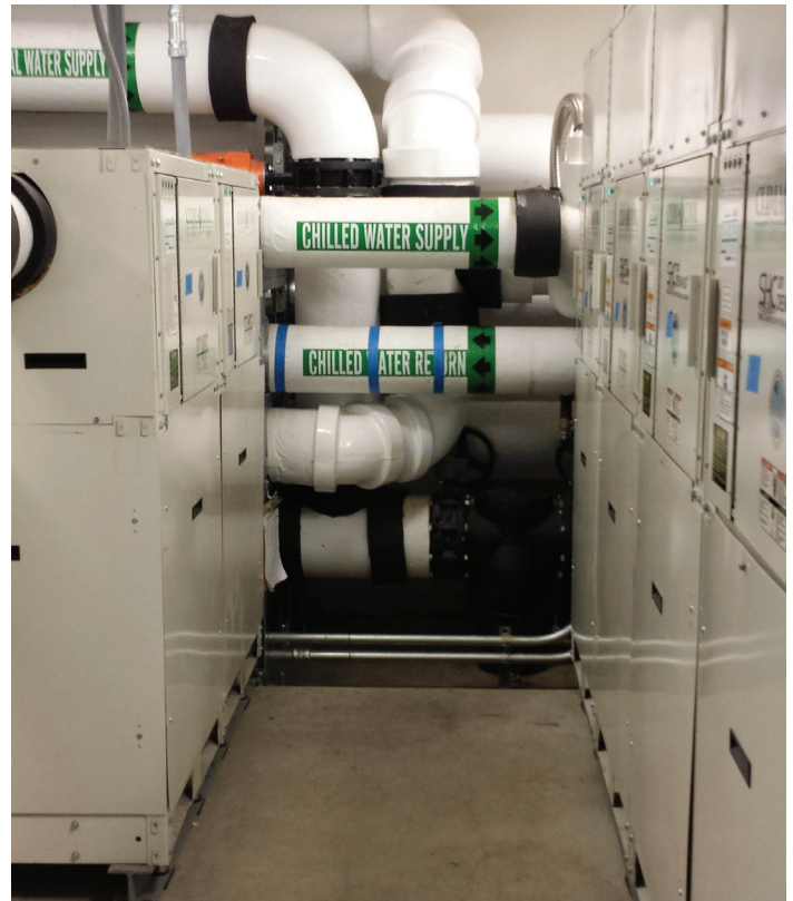
The small physical footprint of the ClimaCool modular chillers allowed the Institute to get additional chillers for increased capacity into the existing space.
