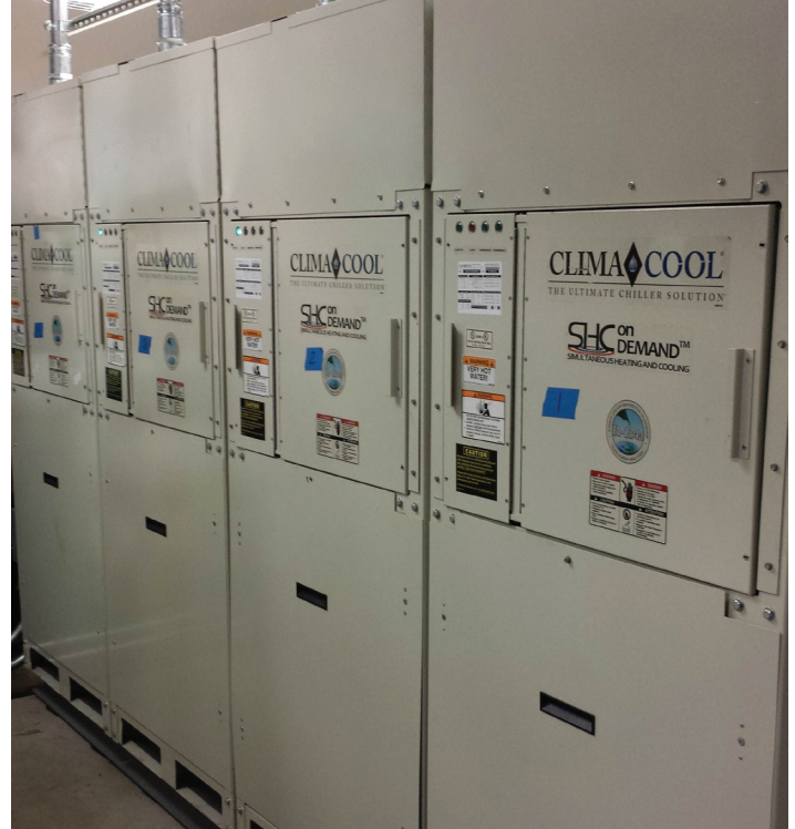
Six modular chillers from ClimaCool, including four 70-ton simultaneous heating and cooling heat recovery chillers and two 70-ton cooling-only chillers, are part of The Buck Institute’s geo-exchange ground loop system.
