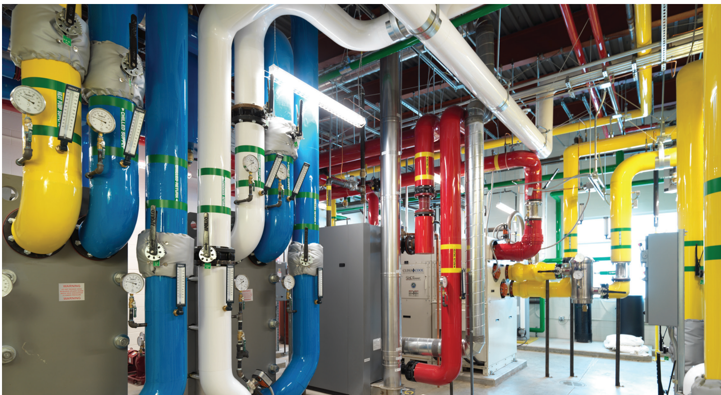
The mechanical room of the Odyssey Elementary school contains some of the equipment comprising the innovative system with indirect evaporative cooling, daylight harvesting, solar panels and a geothermal heating and cooling. The ClimaCool geothermal heat pump is visible in the center.
